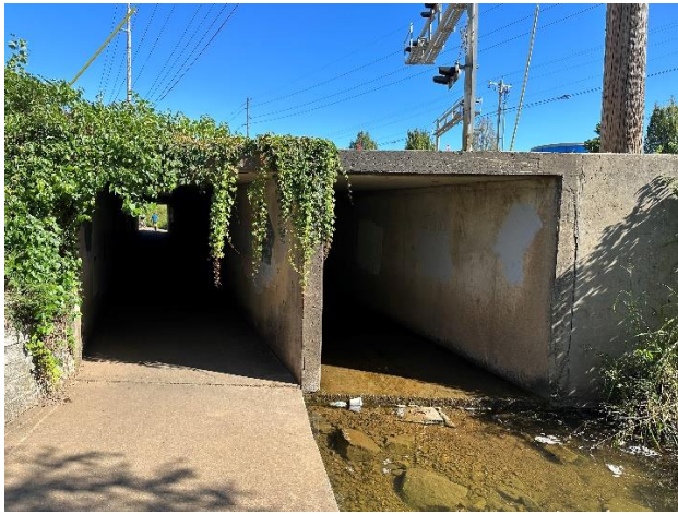
Figure 4: Ex. Underpass at Battlefield Rd.
