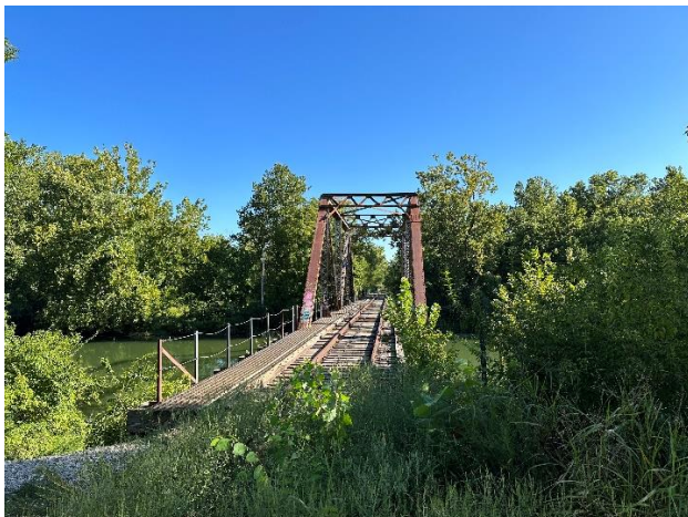
Figure 2: Springfield Lake Bridge
