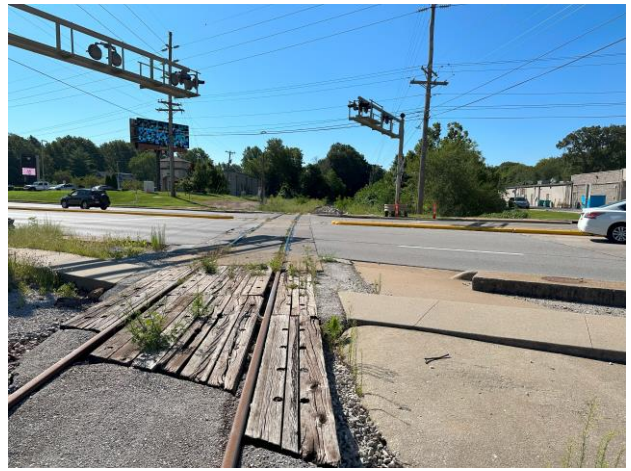
Figure 5: Ex. Rail Crossing at Battlefield Rd.
